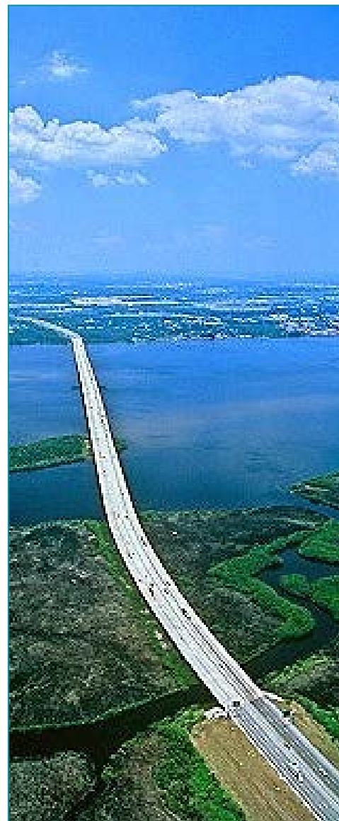
Bridge across the Peace River
